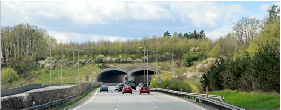
Fig. 3: An ecoduct on the D35 expressway, north of Dolní Újezd.
