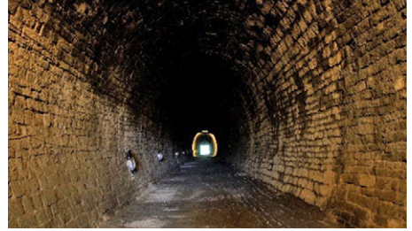
Fig. 5: Abandoned tunnel in Slavíč.
